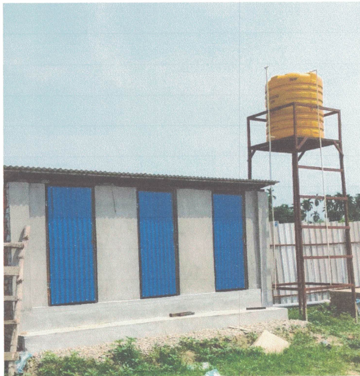
Figure 5. WORKERS TOILET WITH OVERHEAD WATER TANK
