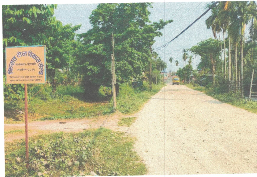
Figure 8. EXISTING CONDITION OF ROAD
