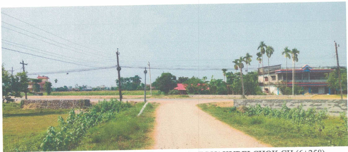
FIGURE-13. END OF ROAD CHAINAGE AT PYAKURELCHOK CH (6+258)
